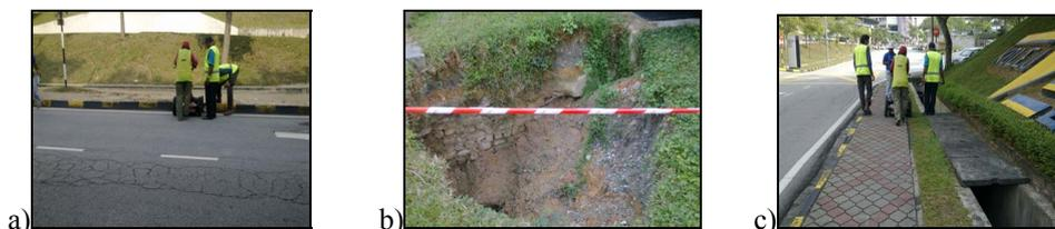
Fig. 3: Site photos. a) cracks on the road, b) sinkhole with depth <7m and c) survey line L1 and L2.
